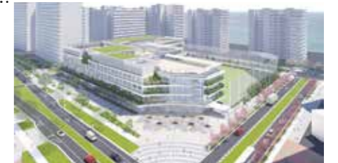
Image of the area at its completion (simulated as of September 2022)
