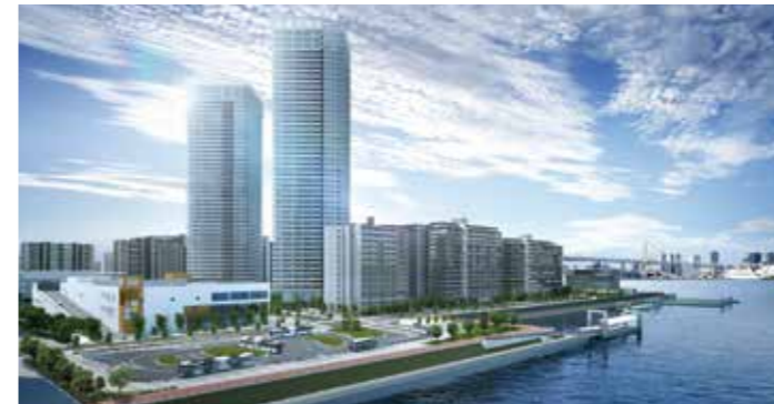
Image of the area at its completion (simulated as of December 2021)
